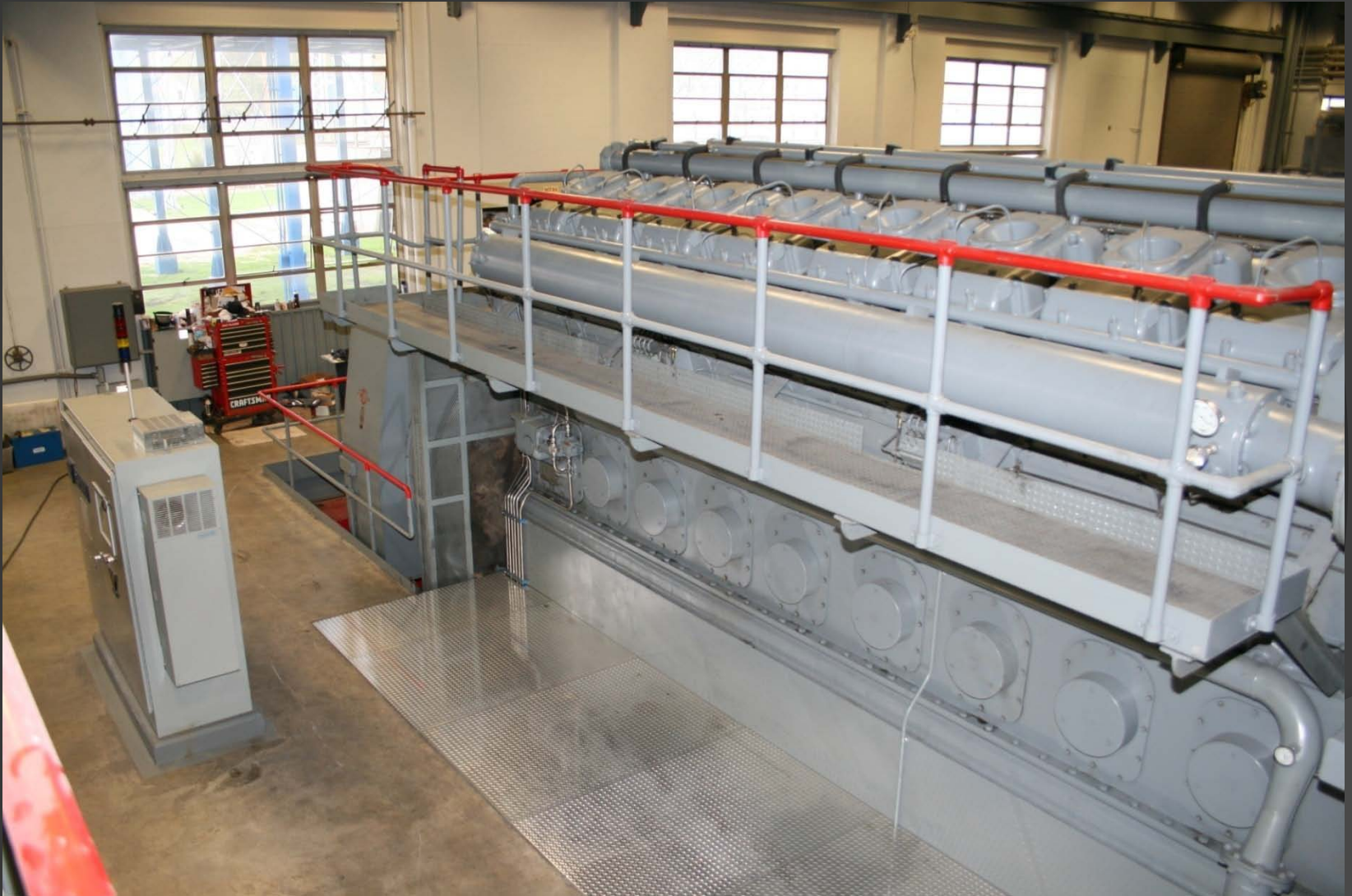
Generator and control panel
