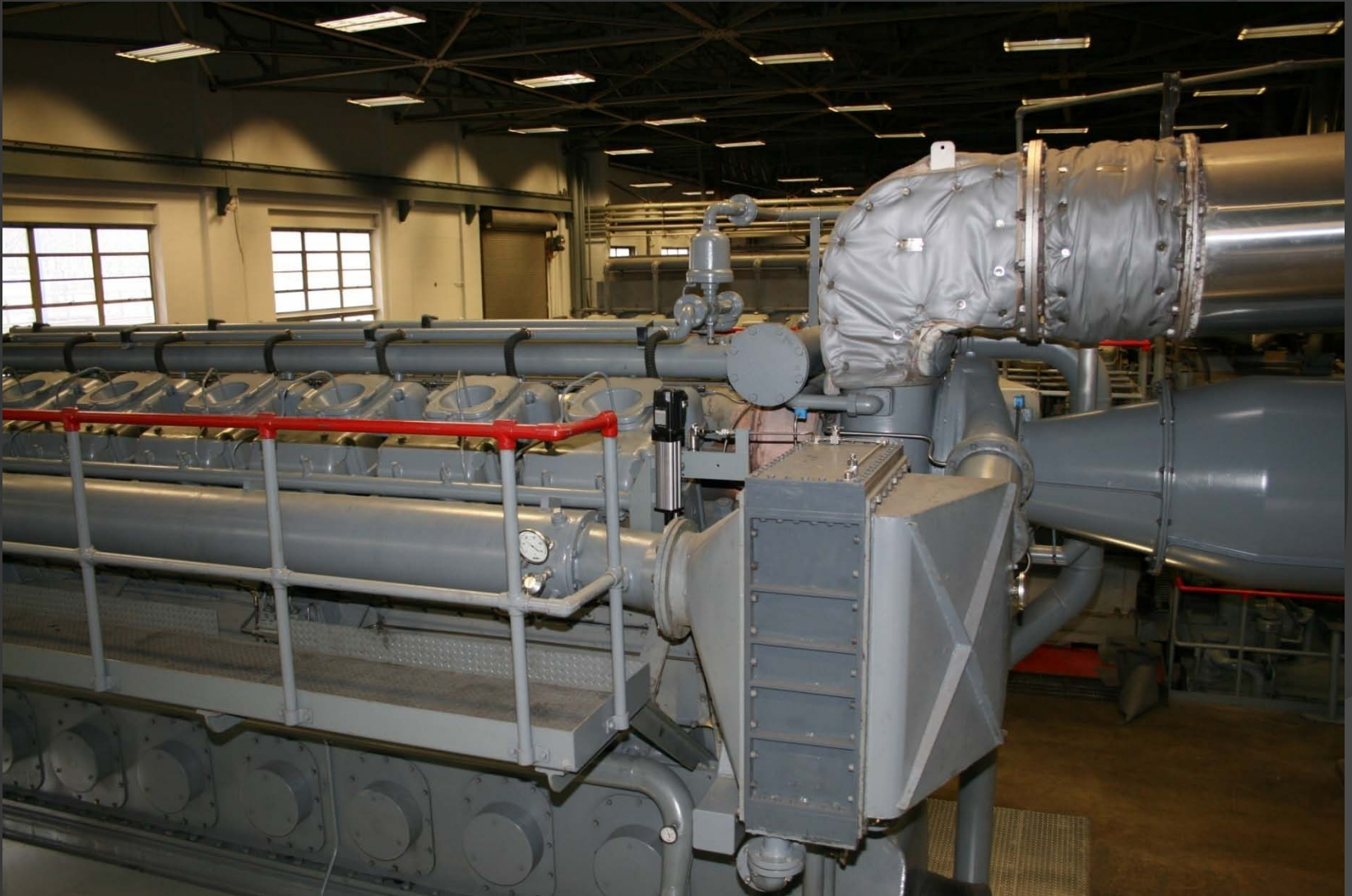
Servo mounted on engine
