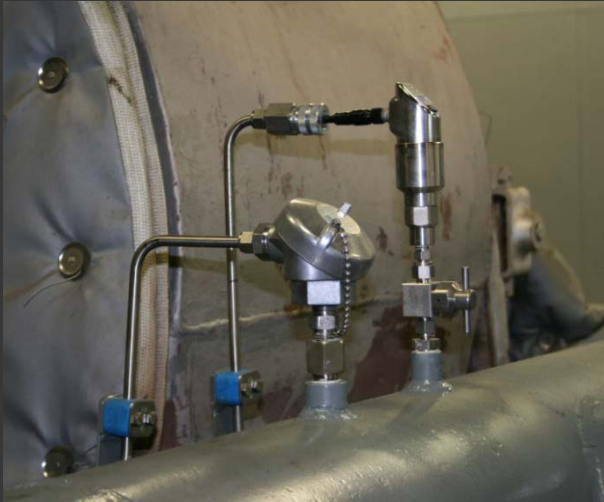
RTD Temperature and pressures
