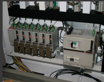
Allen Bradley Kinetix 6000 Servo for governor operations.
