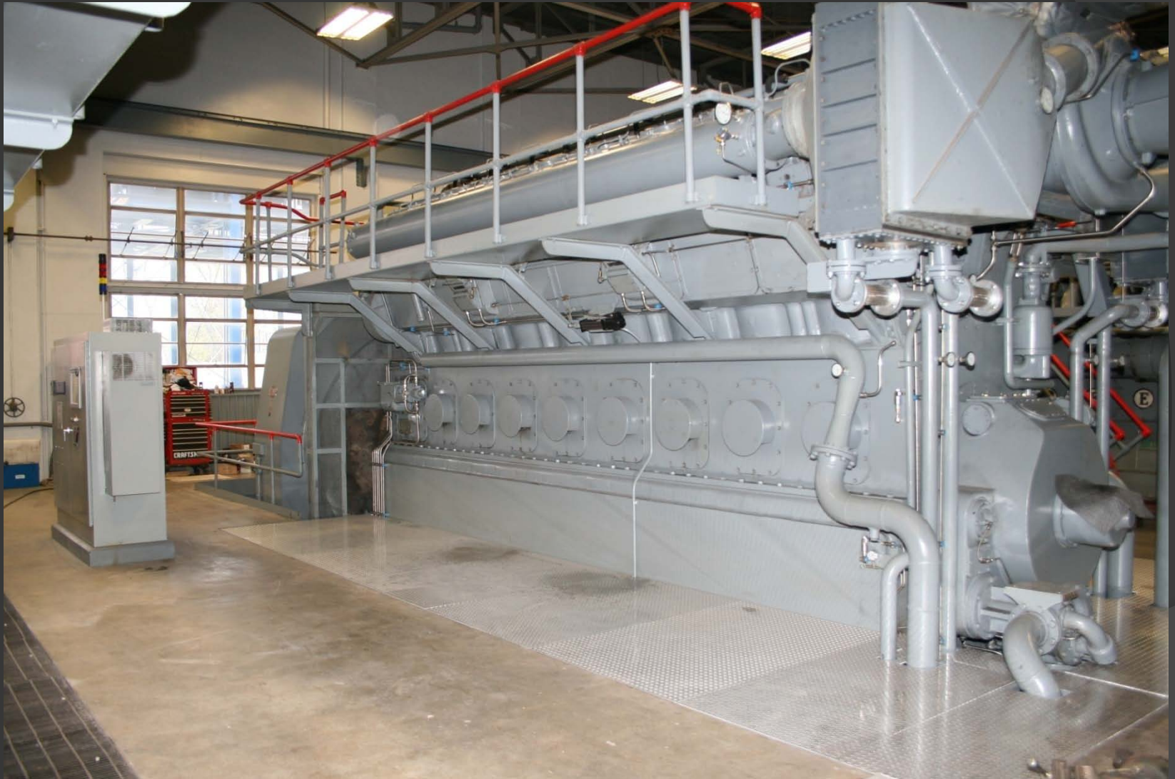
Generator and control panel
