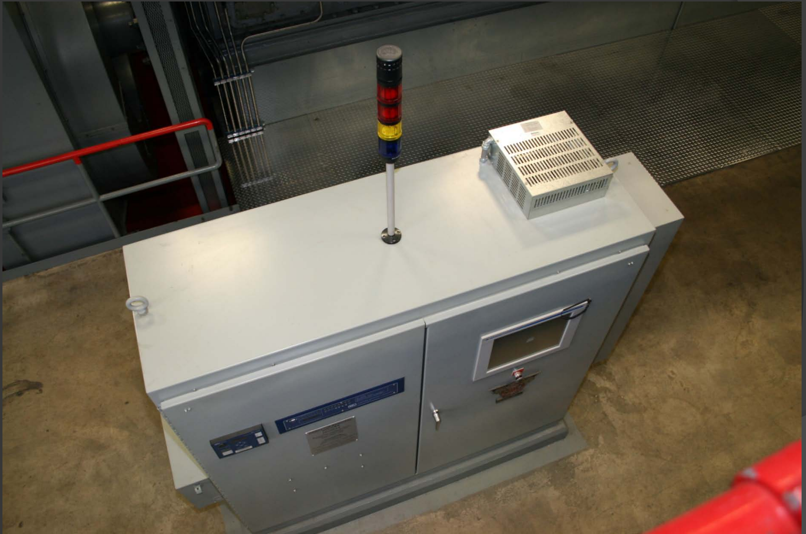
Control panel showing stack light and field resistor cage
