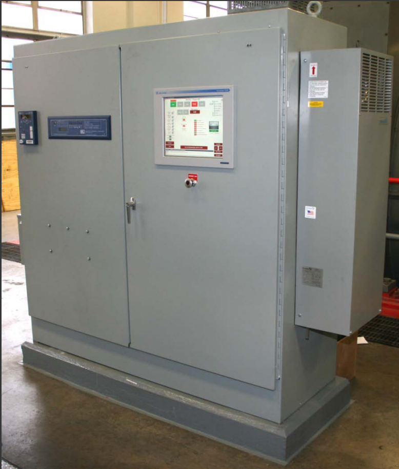
A single air-conditioned enclosure houses the control system and metering / sequence relays. Touch screen operation via Allen Bradley VersaView / RSView FactoryTalk Station .
