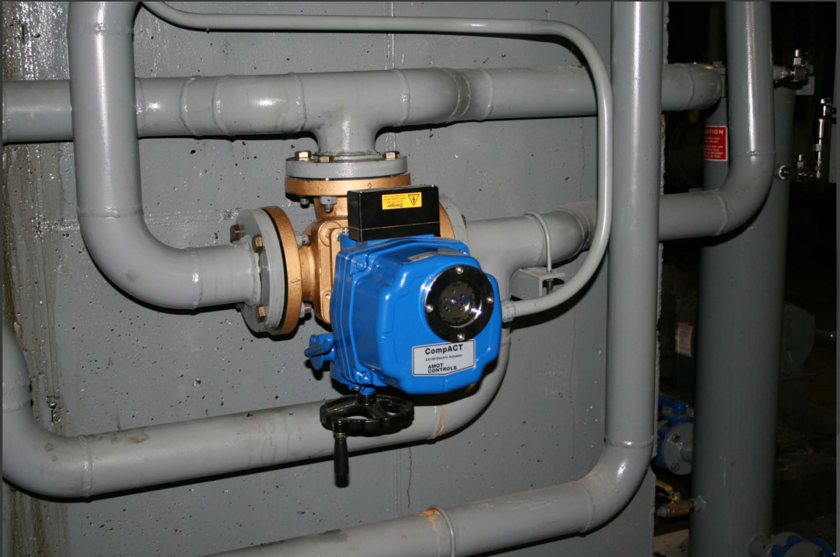
Three-way control valve
