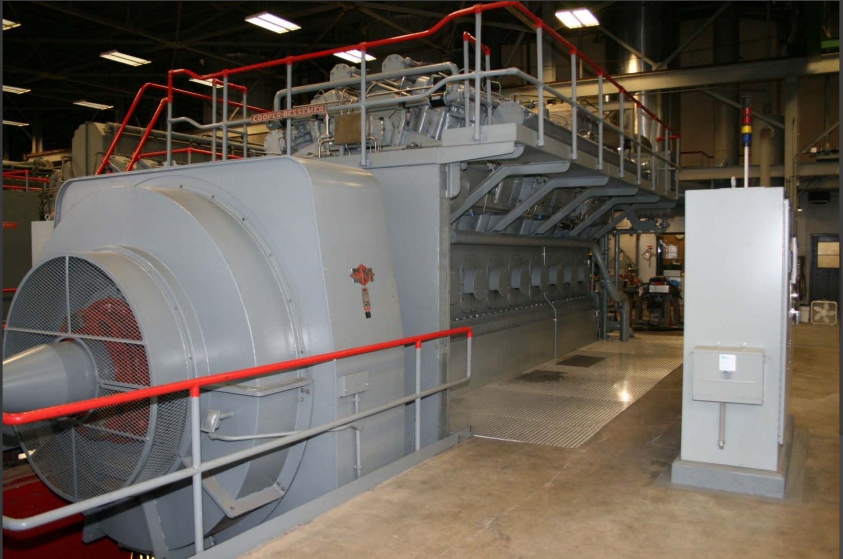
Generator and control panel
