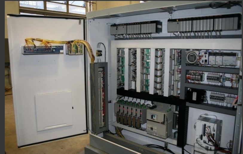
Allen Bradley ControlLogix PLC and support systems.
