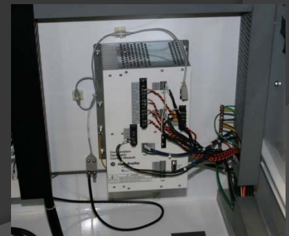
Allen Bradley CGCM for generator excitation and protection.
